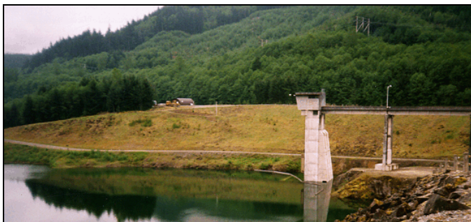
Photo 5-7: Left bank hillside adjacent to the intake tower. The quonset hut storage and staging area is just left of center. May 15, 1998.
