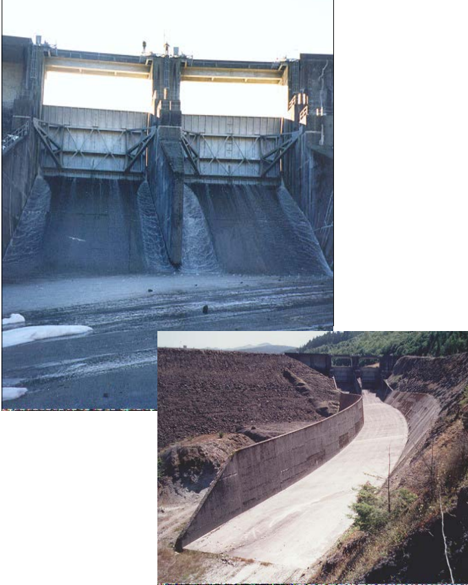
Photo 5-4: Spillway tainter gates (top) and chute (bottom).
