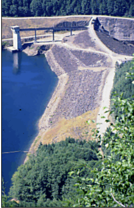
Photo 5-1: Howard Hanson Dam. Intake tower is in the upper left corner with the spillway in the upper right. August 1998.
