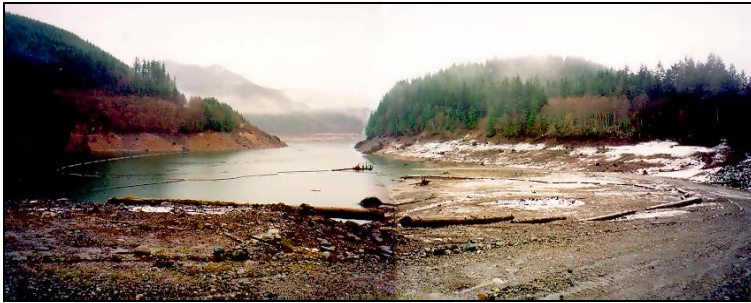
Photo 7-1: The Temporary Debris Storage at the boat moorage area during the winter drawdown at elevation 1,070 feet. Photo shows the crossbooms in place. January 1998.
