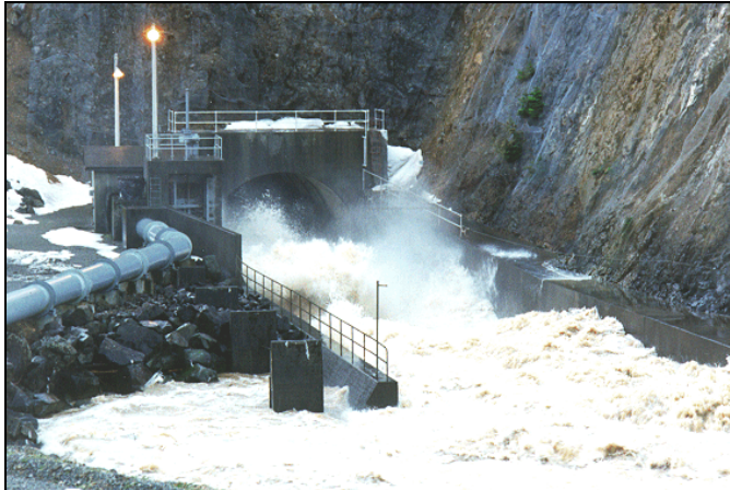
Photo 5-3: Outlet works showing tunnel and stilling basin discharging over 7,200 cfs at 1,183-foot pool, highest pool to date. The 48-inch bypass pipe is located on the left. February 10, 1996.
