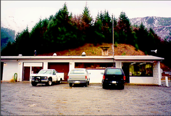
Photo 5-5: Administration building (project office).
