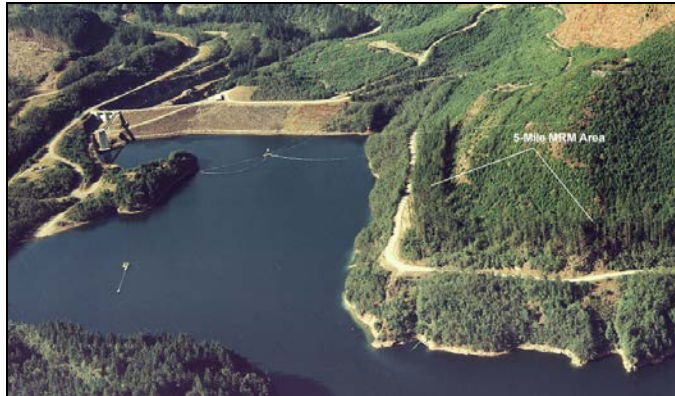
Photo 6-1: The 5-Mile multiple resource management area stabilizes the steep right bank, protecting Road 5500 from mudslides. September 24, 1984.
