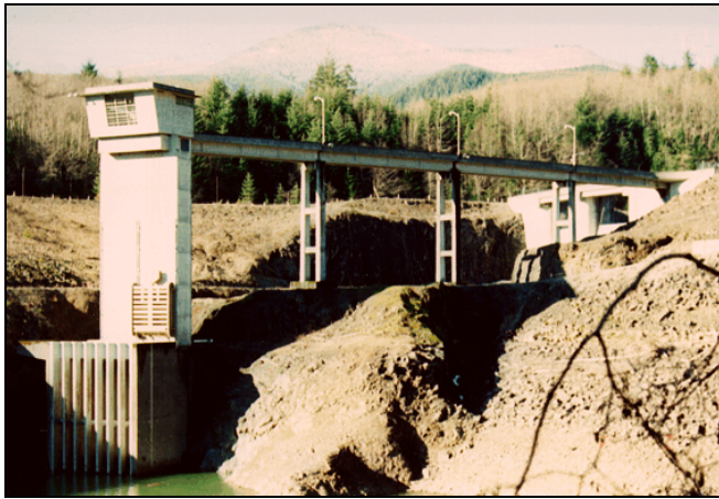
Photo 5-2: Intake tower on the left abutment.
