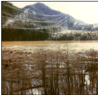
Photo 7-2: The North Fork Debris Storage at elevation 1,177.8 feet. February 9, 1996.
